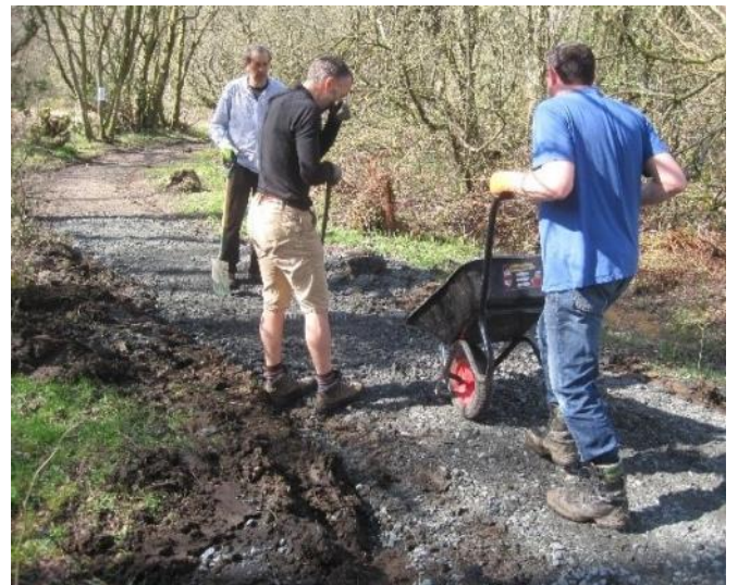
Finishing touches to the path
