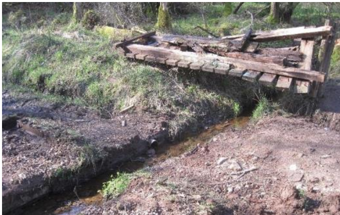
Black Brae Bridge removed
